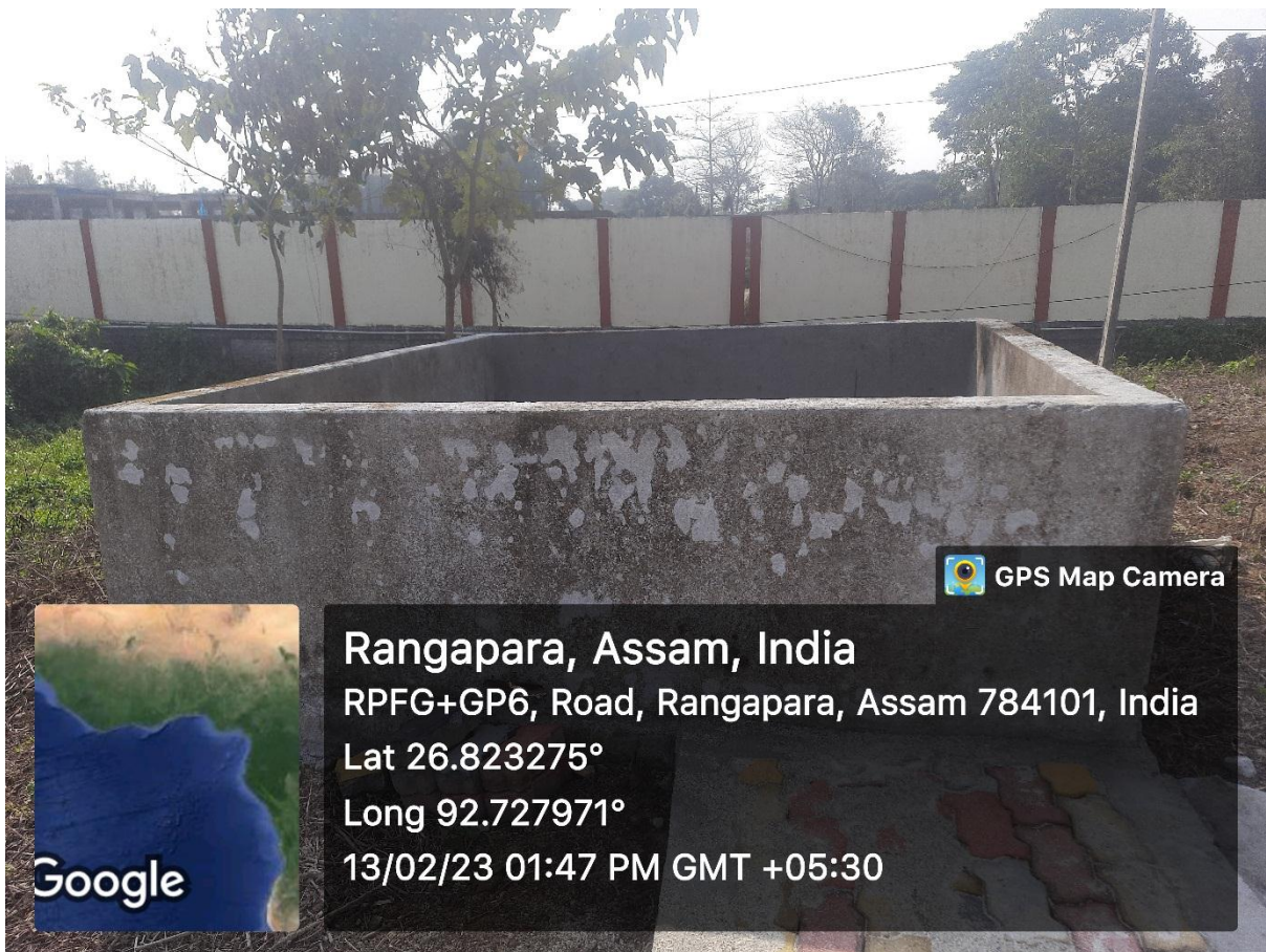
Concrete Waste Disposal Site
